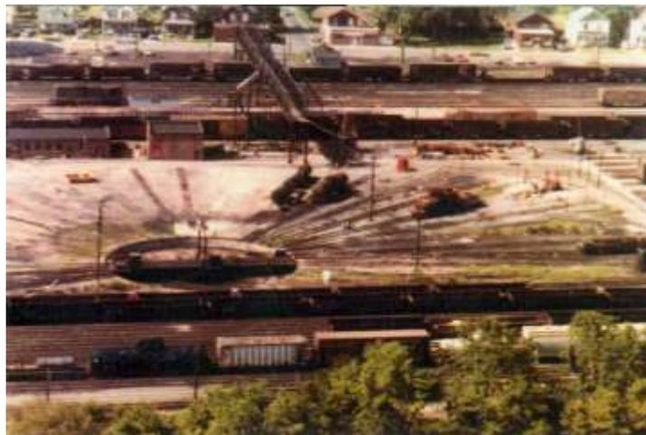
Round Houses were enclosed buildings with track that could turn the Steam Engine around to travel back in the opposite direction.
